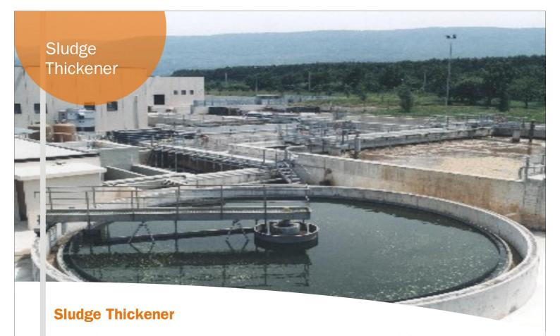
Circular Thickeners provide a crucial treatment step between upstream process screens, clarifiers, and separators and downstream dewatering and sludge conditioning processes. A well-designed thickener provides storage and equalization, reduces the volume of sludge streams, and increases their solids concentrations. This allows for more economically designed dewatering and sludge conditioning systems, reducing capital and maintenance costs.
