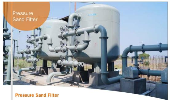
Pressure Sand Filter is used for removal of suspended solids & turbidity from Water & Wastewater. We offer series of filters of different sizes at a low cost, reliable and efficient way to filter your water. It consists of layers of sand and pebbles. Our unique design of Pressure Sand filter ensures the maximum utilization of the surface area, lesser pressure drop across the filter bed and effective removal of the impurities like TSS and Turbidity below 5 PPM and 5 NTU respectively.
